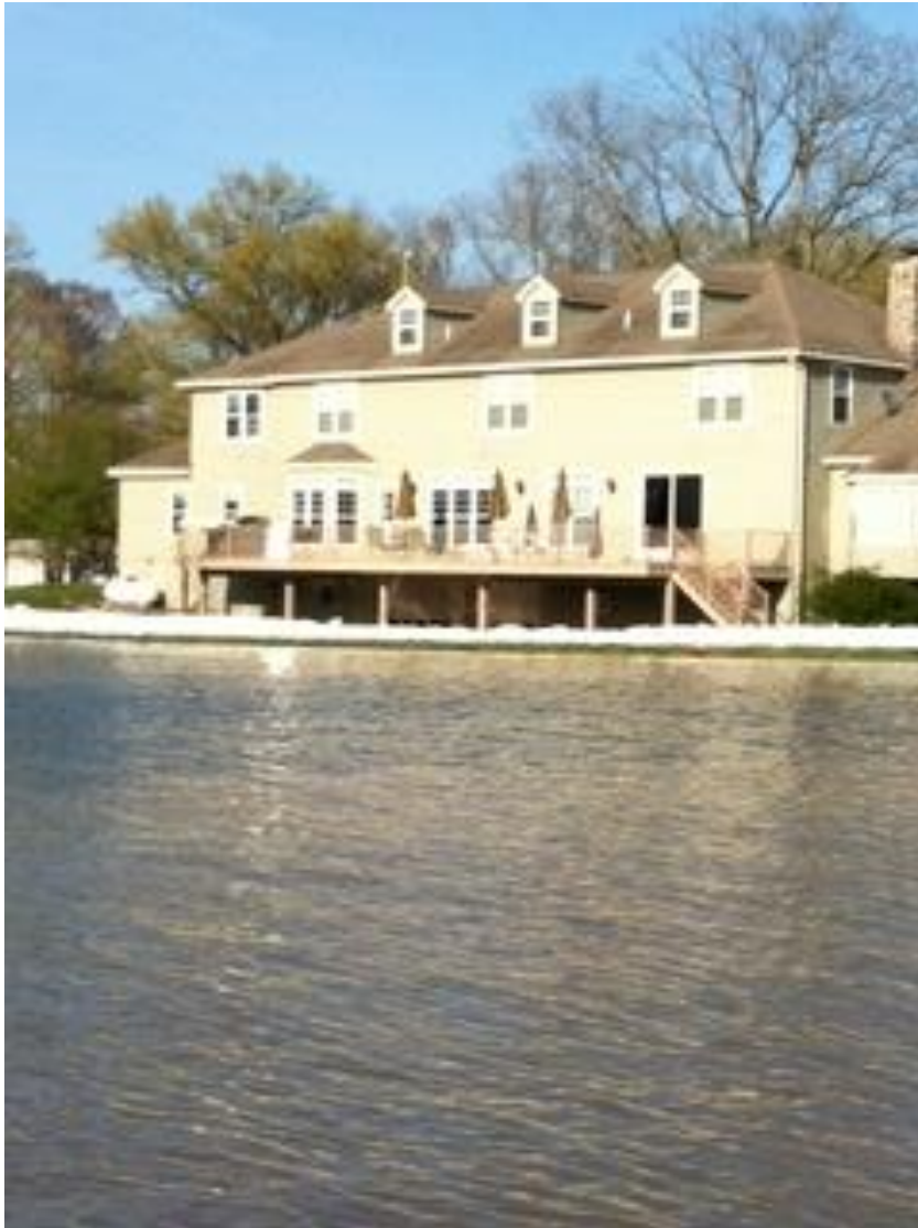
Figure A-5. Floodwaters Surrounding the Clubhouse
