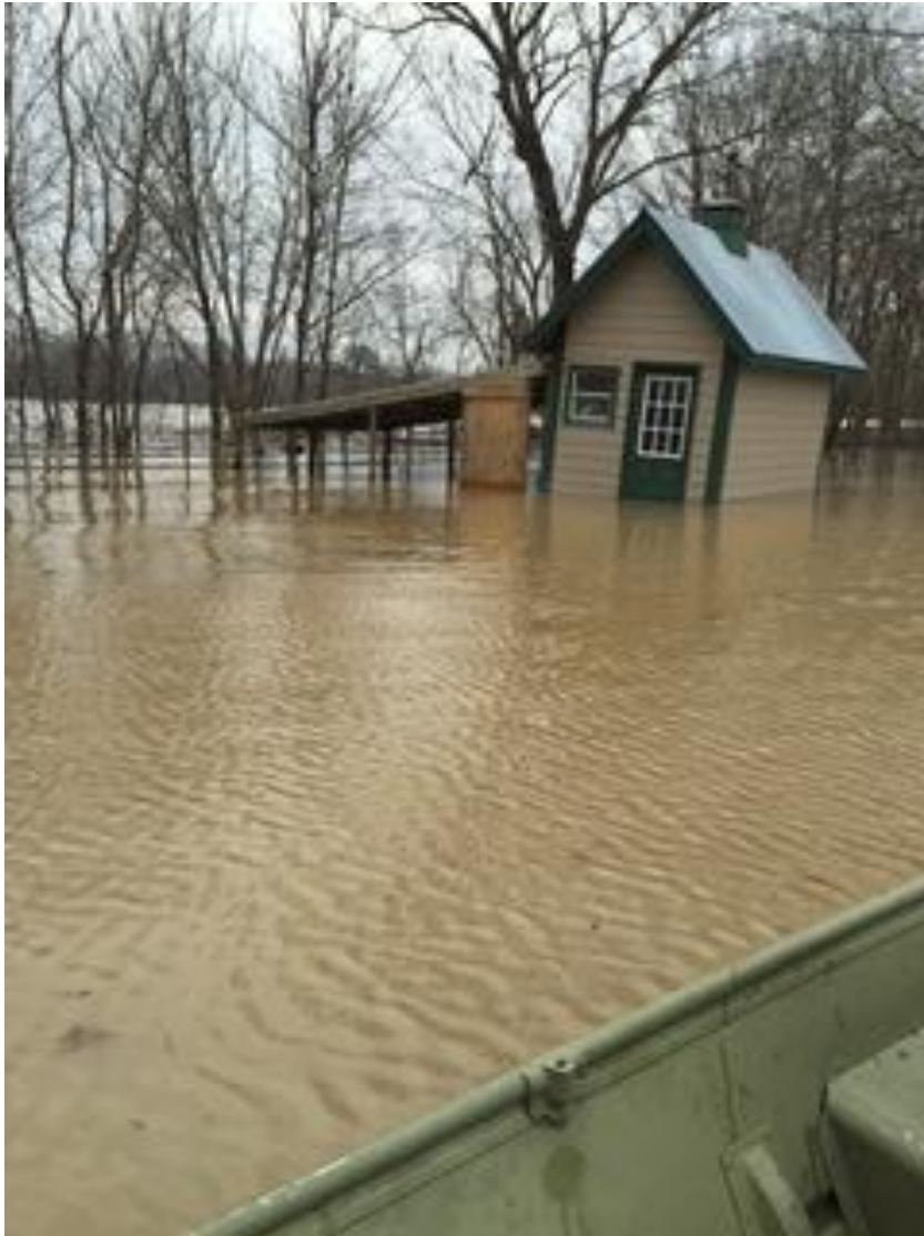
Figure A-14. Flooded Outbuilding
