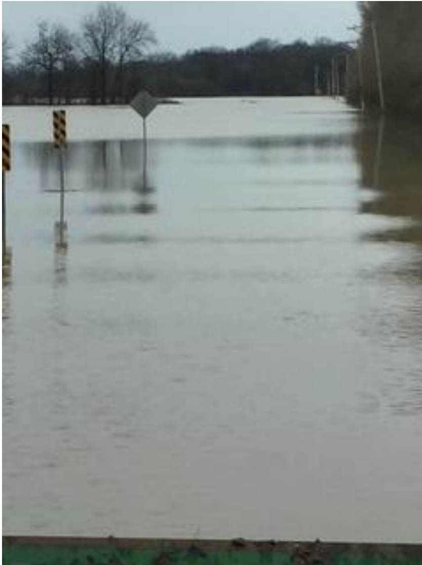
Figure A-12. Flooded Roadway
