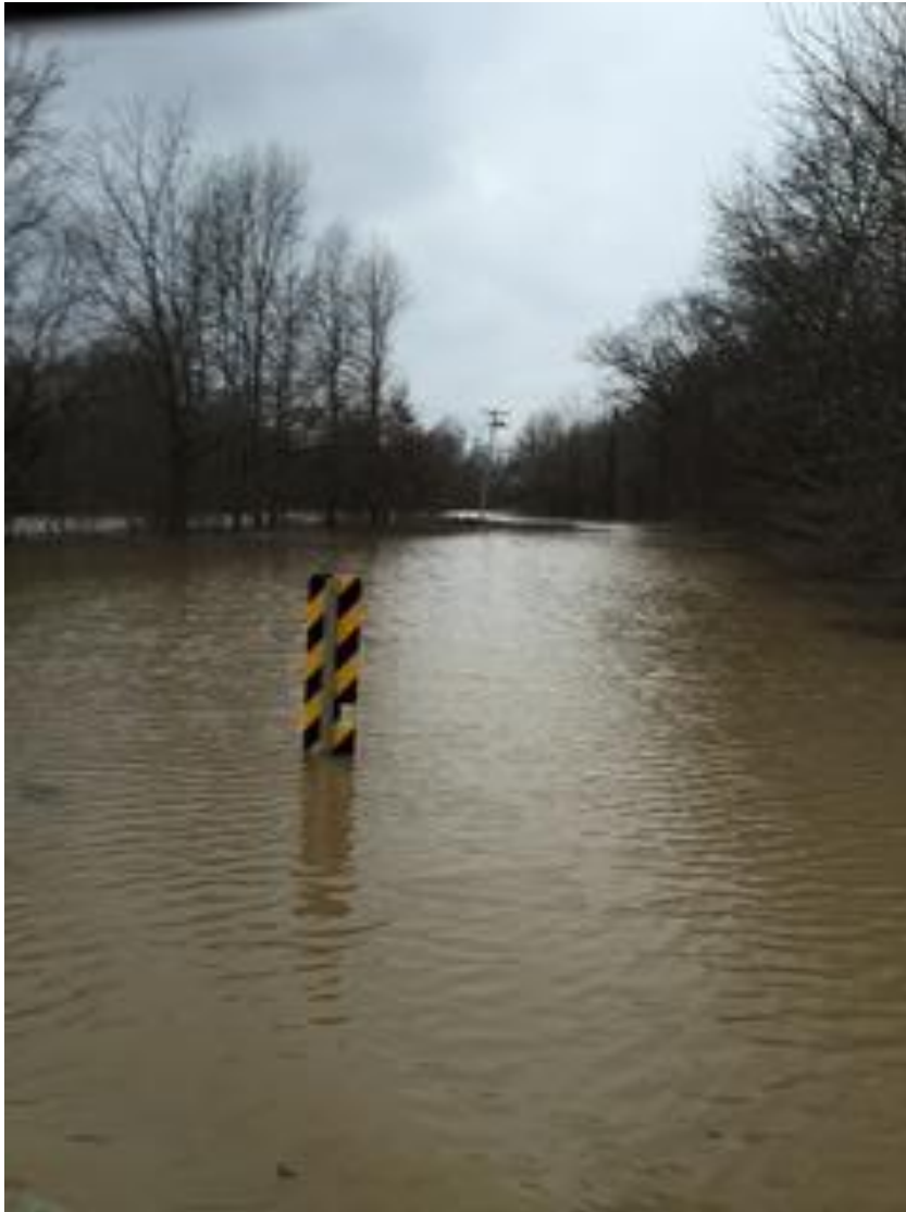
Figure A-16. Flooded Access Road
